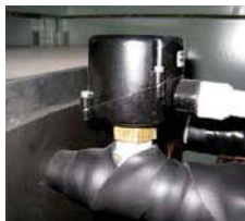
Figure 1 Flow Switch
