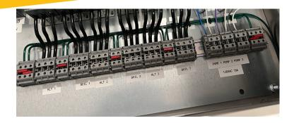
Landing points for electricians to wire to, will be labeled with what they are and torque ratings on the disconnects. For each elemen and pump, landings are available for upto 6 gauge wire for 3 hots, and a convenient ground point.
