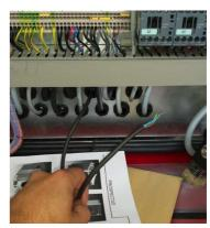
Check the wiring diagram of the chiller appearing at the end of the instruction manual where to connect the cable of the solenoid valve (in this example here the contact inside the control cabinet is X2 -> clips 5, 6 and 7=earth). It doesn't matter whether you connect the brown or the blue cable to clip 5 or 6:
