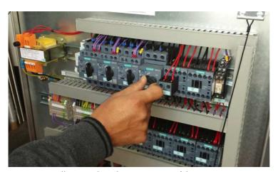
Step 6: Set all circuit breakers to ON = 1 (they are set to OFF = 0 for safety).
